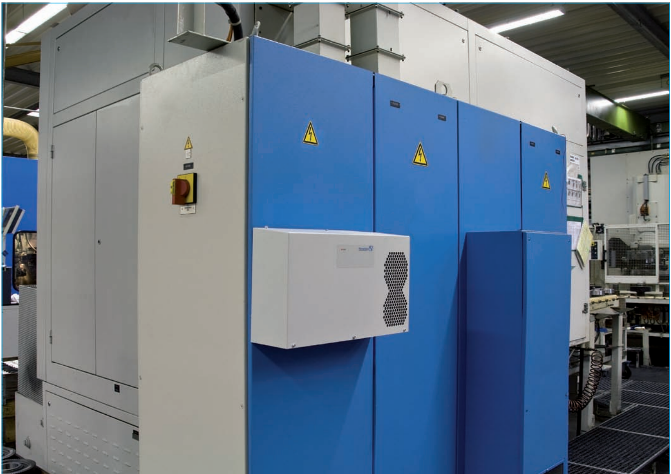
Side mounted cooling units from the Pfannenberg DTS series
